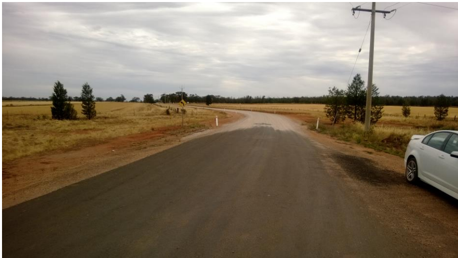
Figure 6 Photo of Cunningham Road from the intersection with The Kidman Way
