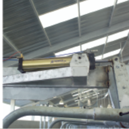
Industrial grade air cylinder — lifts front end of stalls for smooth, rapid exits.
