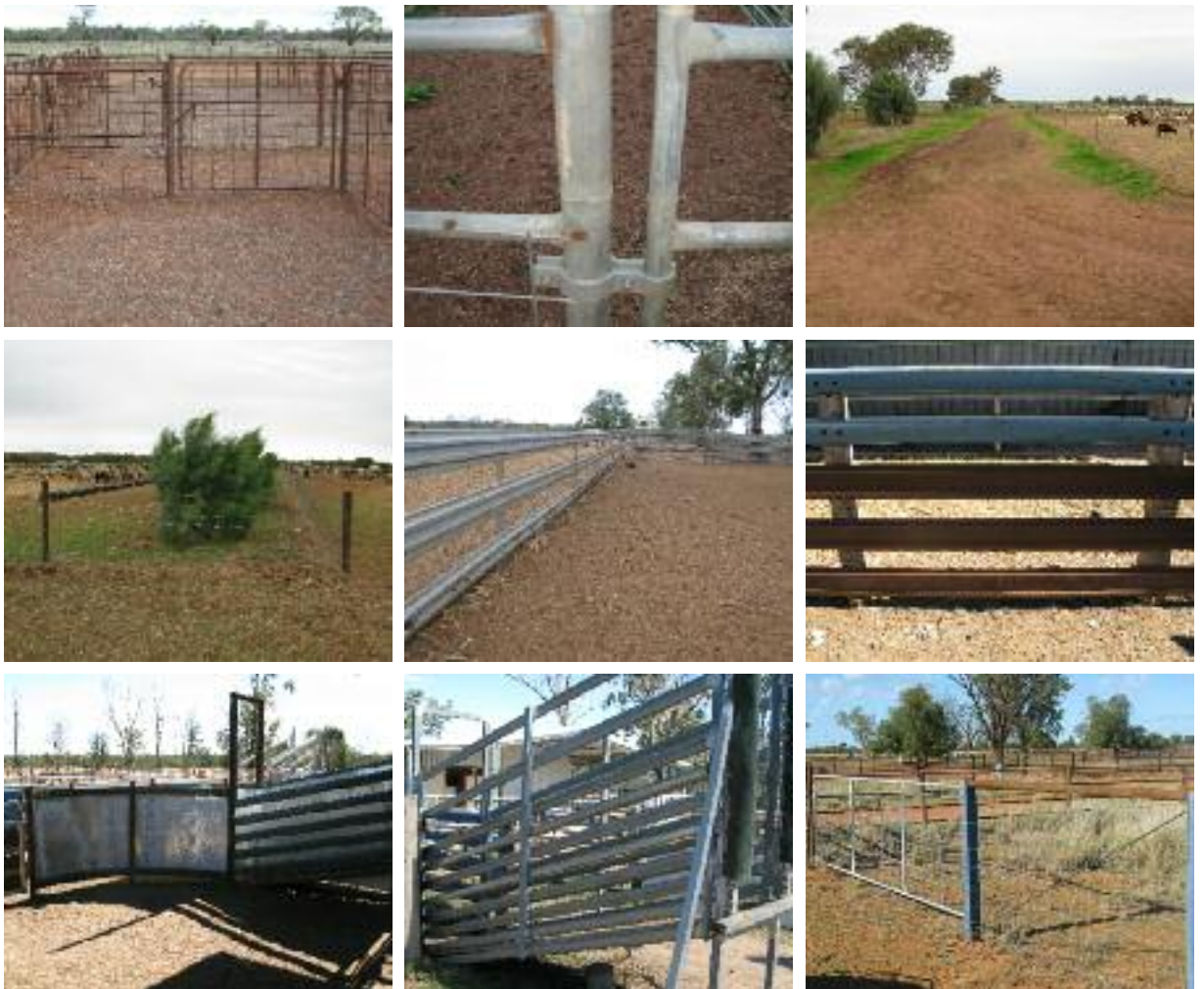
Well-designed and constructed depot yards will improve efficiency and reduce stress
