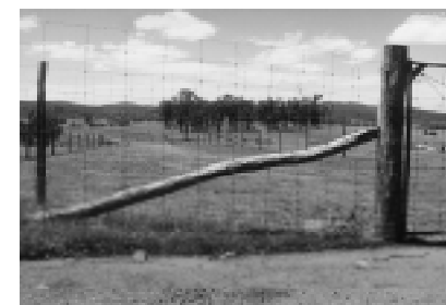
Figure 7: Stay and bed log end assembly
