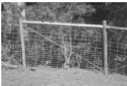
Figure 6: Box style end assembly
