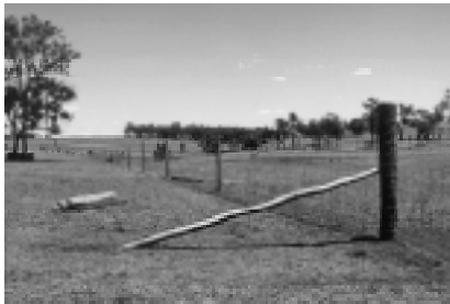
Figure 8: Corner stay (strut and bed log style)
