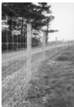
Figure 10: Bed log stay on fence curve
