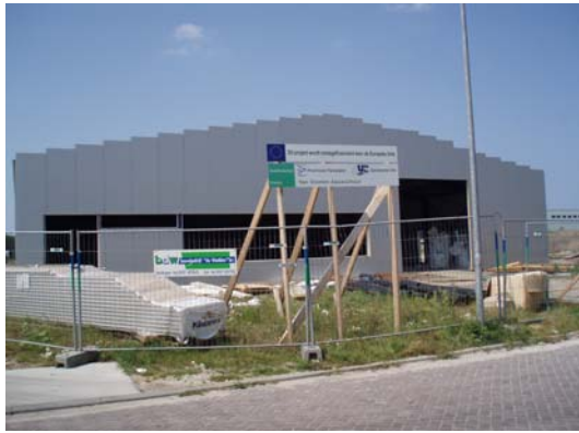
Figure 7.1 The Hesy built recirculating farm for pike perch in Urk, the Netherlands.
