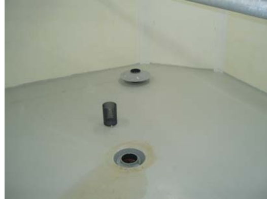
Figure 9.53 One of the large cod growout tanks that had been drained for seasonal maintenance. The Eco-Trap drain is shown disassembled.
