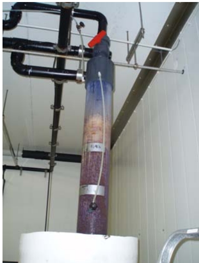
Figure 9.22 A vacuum degassing column was part of the recirculation system for the nursery tanks.
