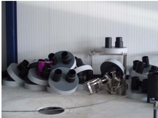
Figure 7.4 Stack of pre-fabricated 'double drains' ready to be installed.
