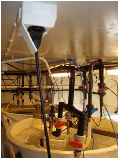
Figure 9.54 One of the rotifer production tanks. The proximity of the electrical outlet (top left) to the tank (less than 500 mm) is of some concern.
