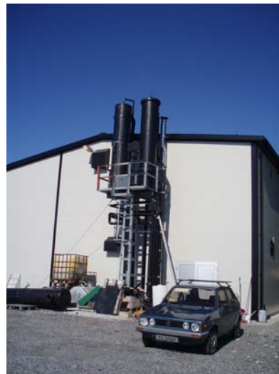
Figure 9.47 Vacuum degassing towers used to treat new sea water.
