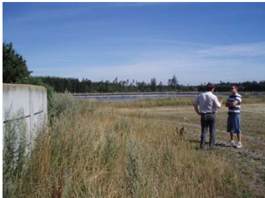
Figure 8.11 The overflow from the settling tank goes to a storage dam (in the distance) and from there it is used for irrigation.
