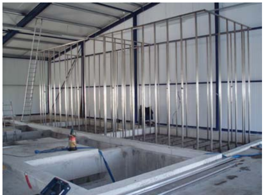
Figure 7.5 The 'skeleton' of the biological trickle filter. The sump in the foreground is designed to hold the drum filter.
