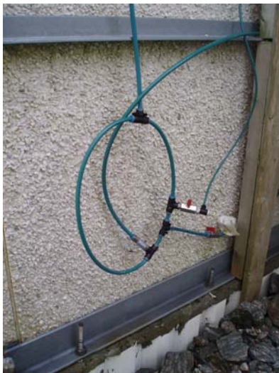
Figure 9.46 'Clip-lock' connectors and plastic oxygen tubing were in use in many of the facilities visited.
