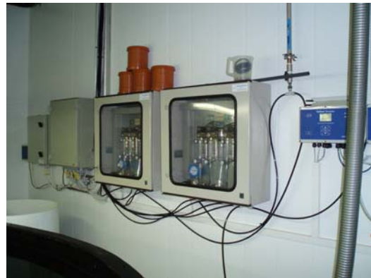
Figure 9.21 This farm also used a centralised oxygen distribution and monitoring station.
