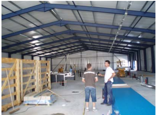
Figure 7.3 Inside the fully insulated shed
