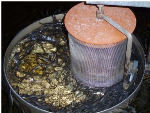
Figure 8.5 A double drain on one of the juvenile tanks. Water from the centre of the tank, upwells to the left of this dish and then passes through the round, self-cleaning, screen and away to the biofilters.
