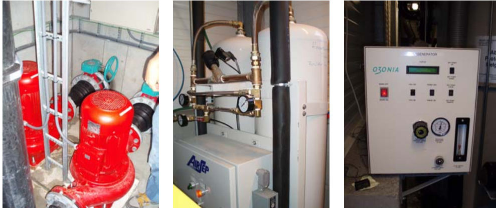
Figure 9.45 Some of the equipment in the Fjord Halibut plant room. L to R, main recirculation pumps; oxygen generator; ozone generator. The problem of not having a floor drain in the bottom of the, below ground level, plant room has recently been overcome.
