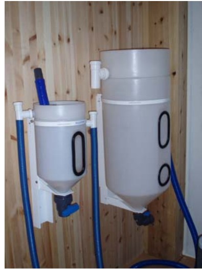
Figure 9.27 The adjustable swirl separators that attach to the Eco-Trap drain.
