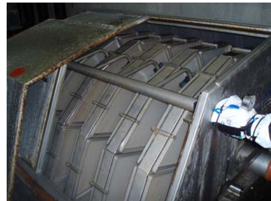
Figure 8.8 The disc filter attached to the main growout system. The discs are removed and pressure cleaned every two weeks.
