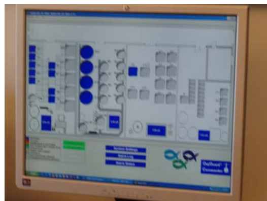
Figure 8.22 All the tanks in the centre were mapped on the computer based oxygen monitoring system.
