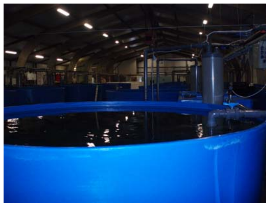
Figure 7.10 Inside the shed. The former chicken shed has been refitted as a fish farm. The tanks are all high density HDPE and there are 16 'cells' each containing 2 x 10 000 litre and 1 x 4000 litre tanks. The shed is dimly lit to less than 150 lux.
