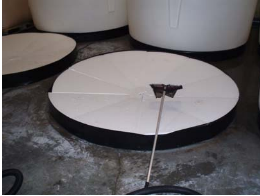
Figure 7.13 The bases of the culture tanks are made from wedge shaped pieces of polystyrene.
