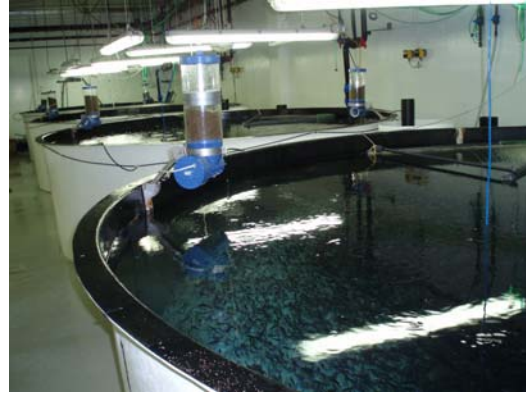
Figure 9.25 Part of the cod nursery. Each tank was serviced by a small Arvo Tek automatic feeder.
