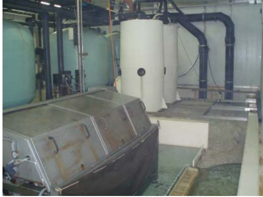
Figure 9.24 The main sump, sand filters and degassing area for the recirculation system. This was considered to be 'old' technology.
