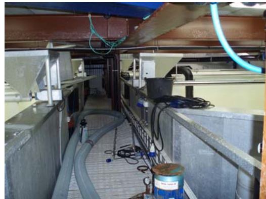
Figure 9.55 Walkway between the tanks in the growout area of the farm. One of the problems of retrofitting an old building as a fish farm can be seen in this photo...note the overhead beams and lack of head clearance.
