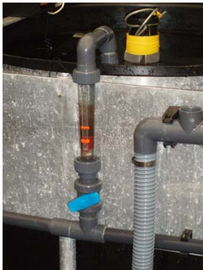
Figure 9.6 Plastic flow gauges were in use throughout the facility and appeared to be more robust than the plastic gauges with metal flow indicators that have previously been on offer in Australia.
