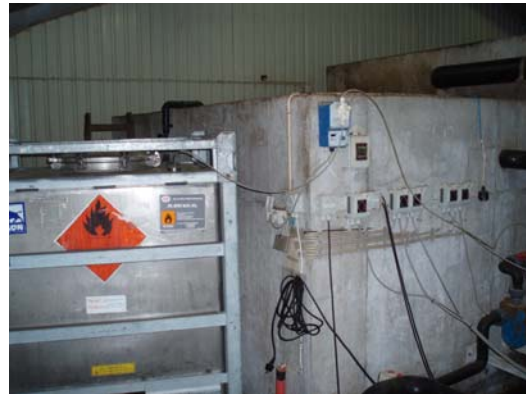
Figure 8.12 The nitrate concentration of the recirculated water is reduced by passing some of the flow through a denitrification tank, which is supplied with alcohol to drive the process.
