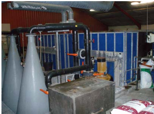
Figure 8.7 The recirculating system attached to the juvenile tanks. The blue 'box' at the back is the trickle filter and the oxygen cones are to the left.
