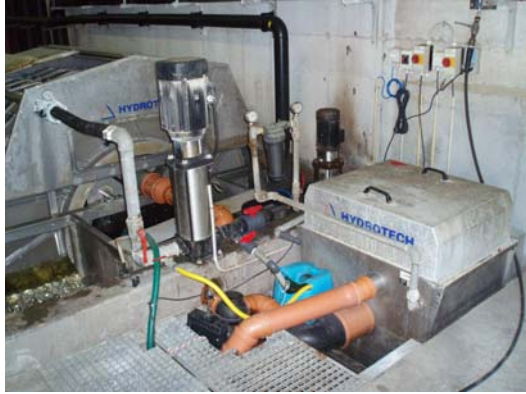
Figure 8.9 The small drum filter attached to the backwash stream of the disc filter. This filter further concentrates the solid waste before it goes outside to a settling tank.
