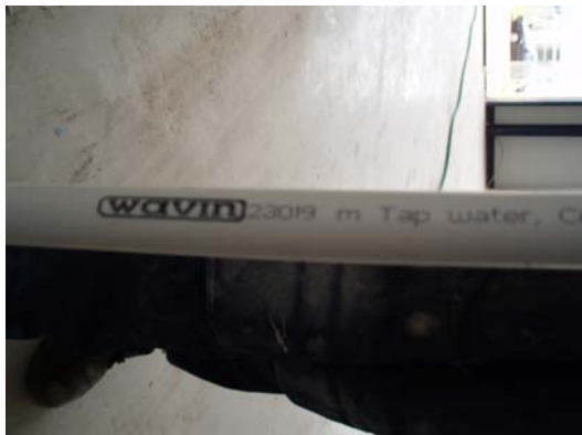
Figure 7.6 The flexible piping used to reticulate oxygen around the shed. Much more cost effective than copper.
