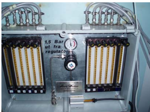
Figure 9.12 All oxygen controls for the larval rearing system are in one, easily accessed panel.
