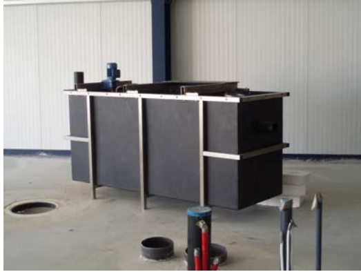
Figure 7.7 The polymer mixing tank. Effluent water from the drum filter is pumped into this tank, mixed and then the flocculant goes to the belt filter.
