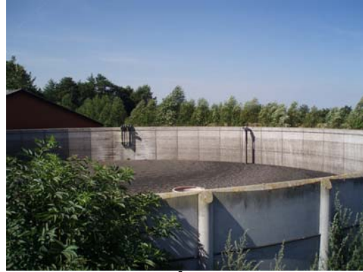
Figure 8.10 The 600 m 3 outdoor settling tank.
