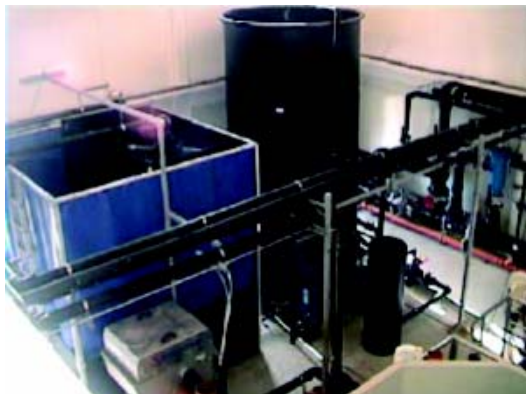
Figure 9.50 The AquaOptima designed bio towers and recirculation system
