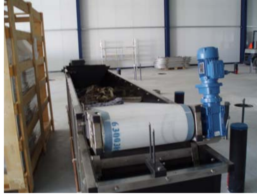
Figure 7.8 The belt filter, just out of the box and ready to be installed.
